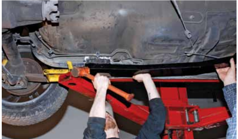
> The chassis makeover began with the installation of a pair of Hotchkis subframe connectors. To obtain a good fit and a solid basis for welding, old paint and sealant were ground off the mounting areas on the rear pan rails and front subframe.
