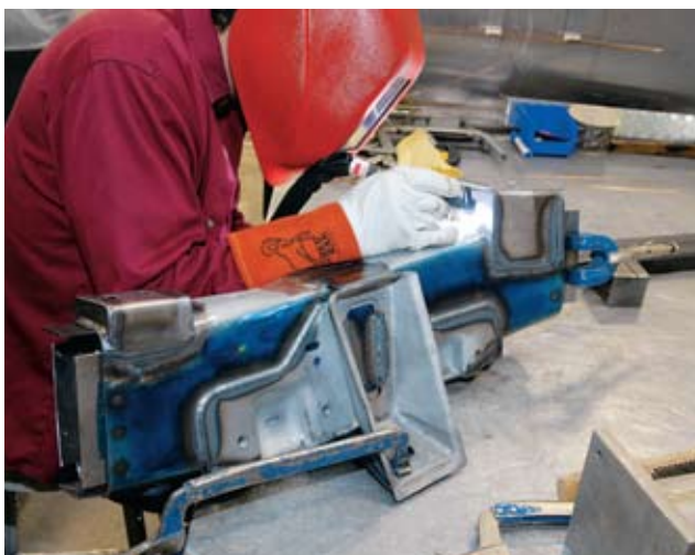
The stock Corvette framerrails have been cut and will be grafted with the '57 frame. Here, you can see the roll welds on the Corvette frame with mounting plates. Four-inch plates extend 2 inches into each side of the frame.
